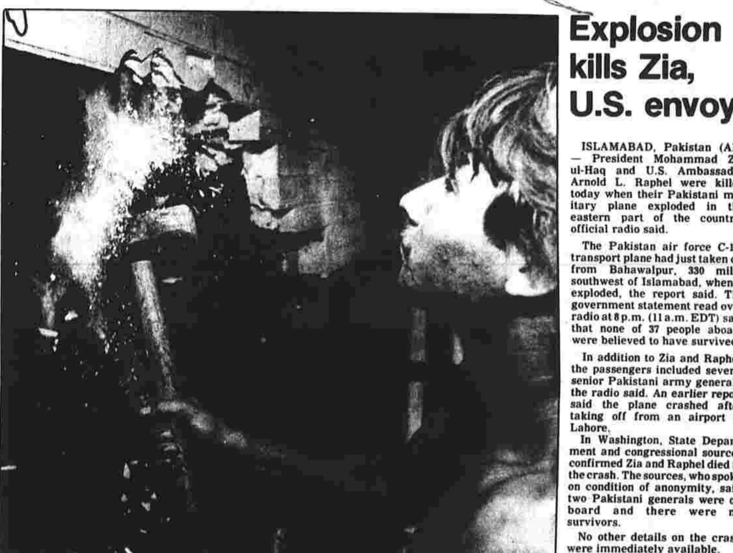
WALL WORK — Ken Dottle of LaRose Construction works to knock down a wall in the cafeteria at Bowers School on Tuesday.
